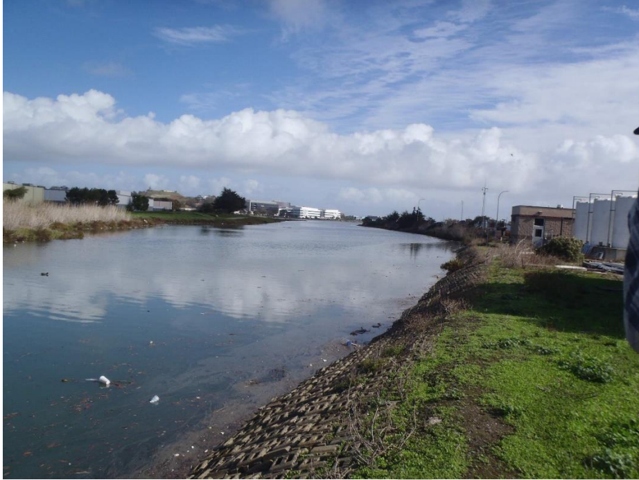
Figure 3. North floodwall alignment view east of Colma Creek, articulated concrete mattress.
