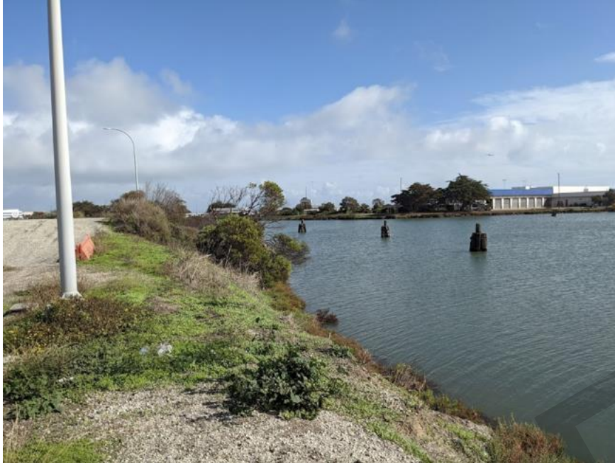
Figure 5. View west of south floodwall alignment east end (furnished by Corps of Engineers).
