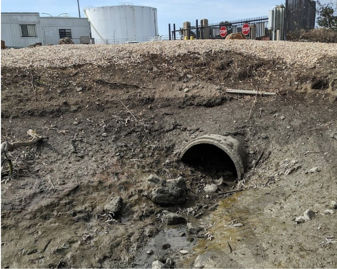
Figure 4. Stormwater outfall that crosses wall alignment and is inundated at high tide.
